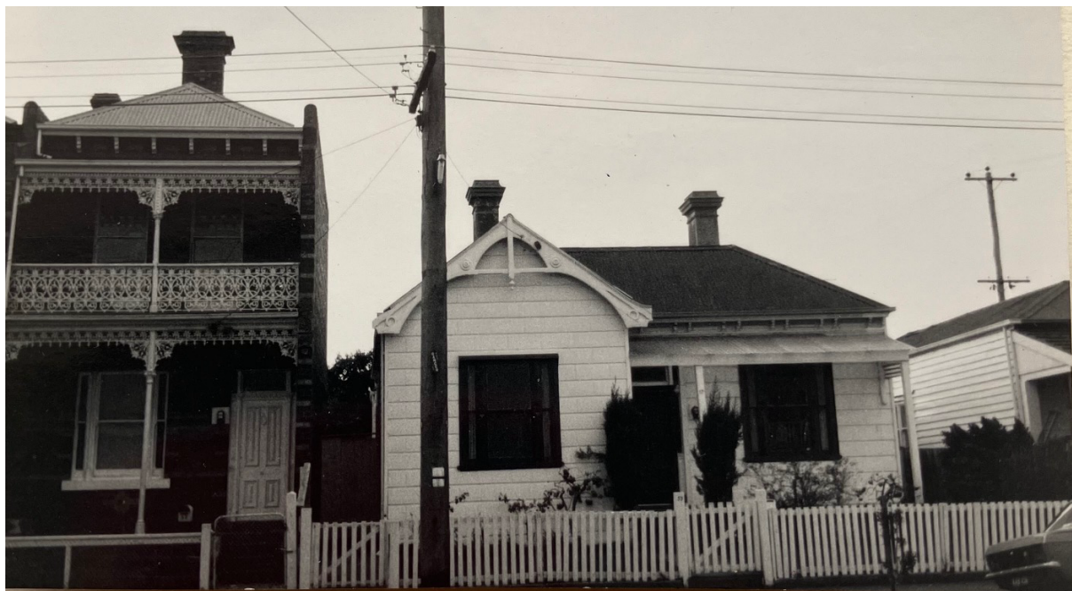
Roseneath Street 1974: Our house with Peace and Prosperity by the front steps and the new street tree
